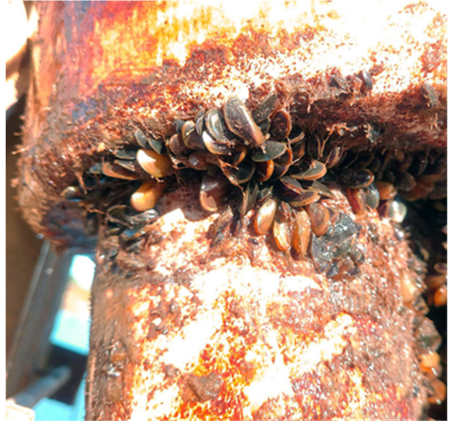
DWR monitoring equipment. Oct 2024.
